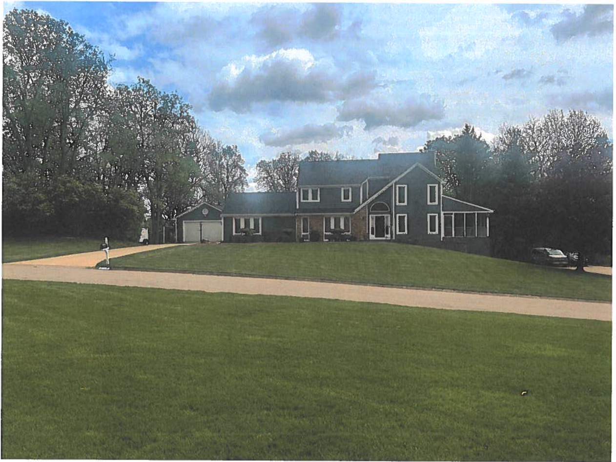
7775 Glen Eden Lane, across the street, with one story garage addition at the side
