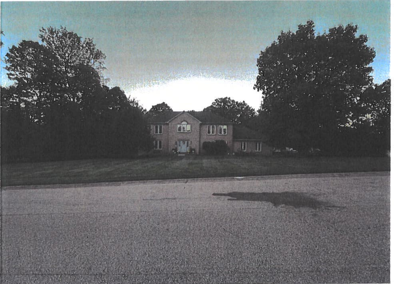
View from Street, Facing West, Proposed Location of Granny Cottage is minimally visible from this location, will be behind the parked cars at the right in the photo
